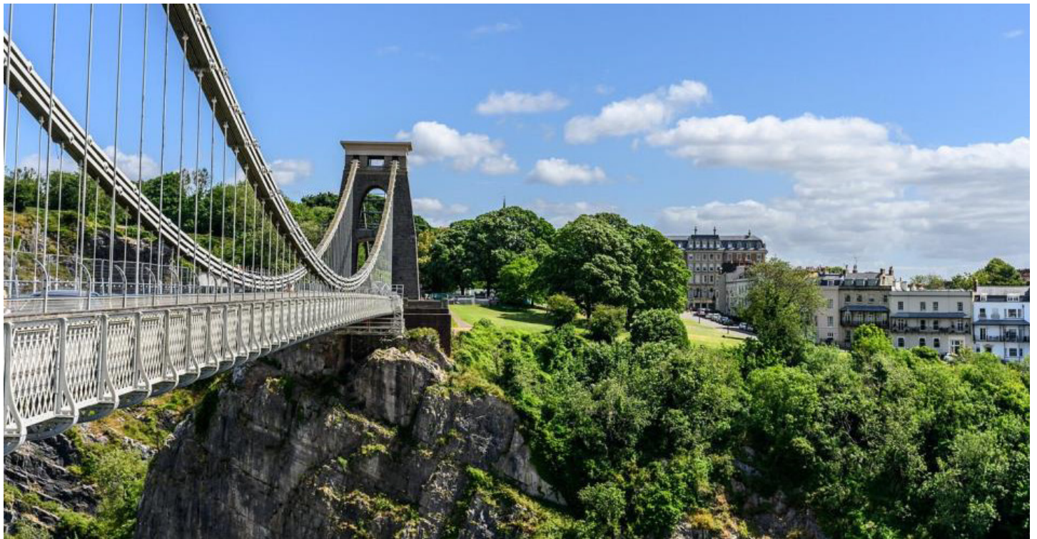
The famous Clifton Suspension Bridge over the Avon Gorge, which you can visit on a heritage coach trip © Clifton Suspension Bridge Museum
